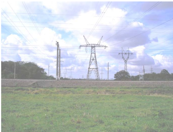
Fig. 3. Transmission lines crossing the railway track
